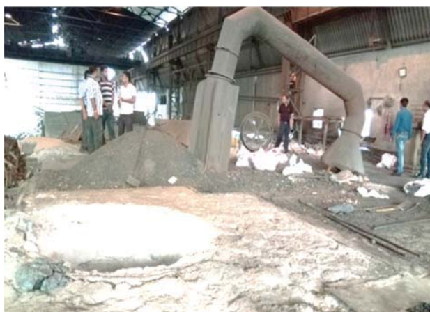
Fig. No.3.4: Pollution control device in dilapidated condition in M/s. K B Sponge Iron Limited
