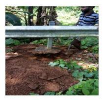
• In four completed works having provision for W/Thrie-beam metal crash barriers, adequate quantity of cement concrete was not provided for fixing the vertical posts as required by the specifications as detailed in **Table 3.1.2**, which was confirmed after excavation around the vertical posts in the presence of Departmental officers. This indicated failure in supervision by Departmental authorities.
