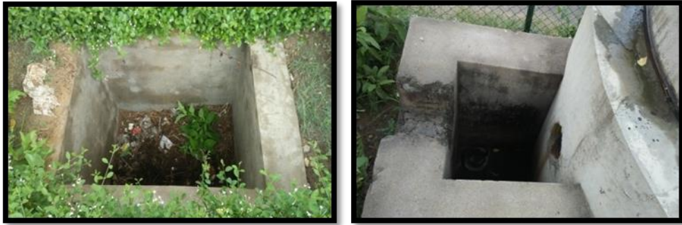
Non-functional Rain Water Harvesting pits
