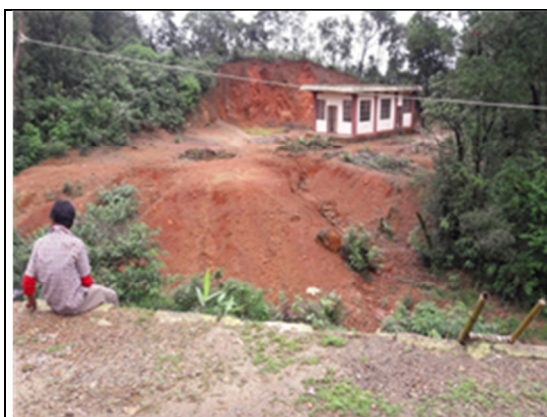
Photograph – 2.2.3 Unutilised community halls at Mawbeh village.
