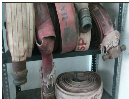
Pictures 5 and 6 : Worn out water hoses
