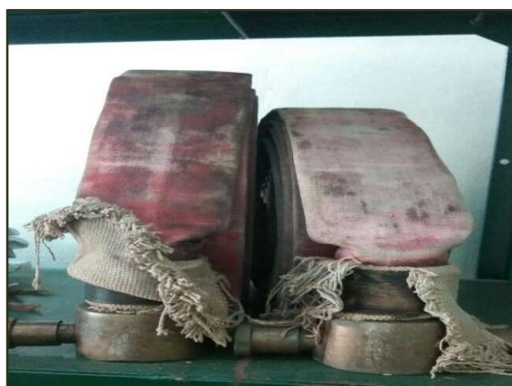
Pictures 5 and 6 : Worn out water hoses
