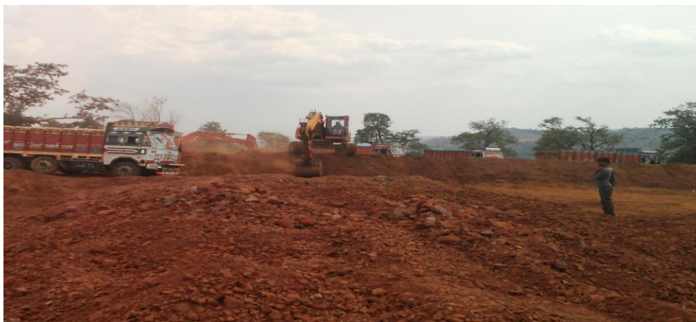
(Bauxite mining at Daldali mine in District Kabirdham)
