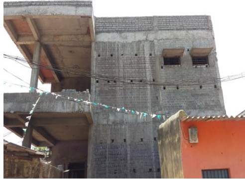
(Incomplete zone office building at Raigarh town)
