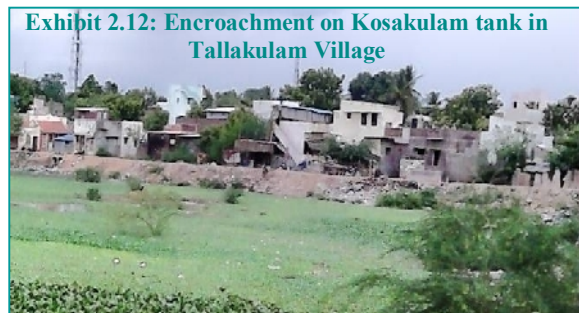
(Source: Photos taken during joint inspection)
