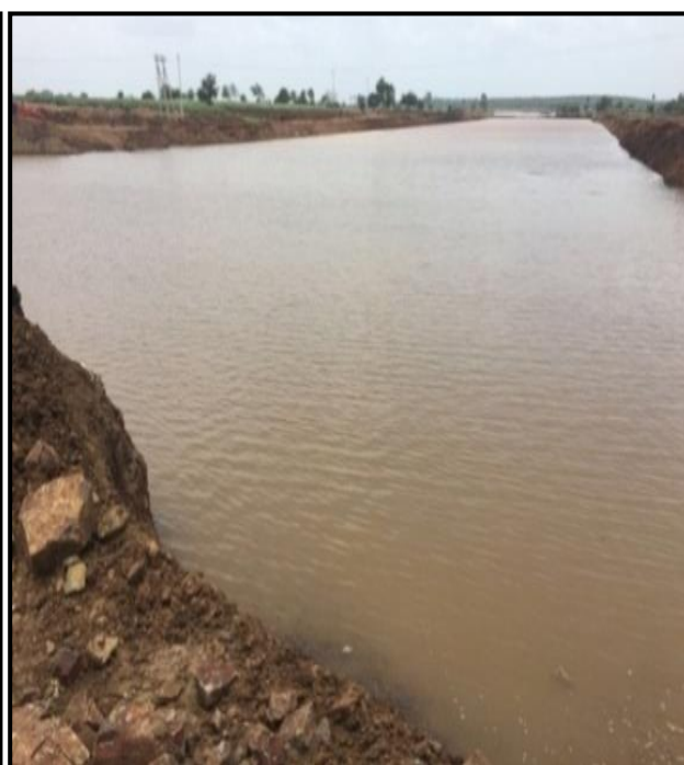
Chart No.2.1.4: Intake channel after submergence when water was beyond RL 507 metres (July 2016)
