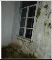
Walls inside the MO's quarters of Nonglang PHC is damp and partially damaged due to leakage of water
