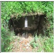
A toilet in the premises of Shallang PHC drains into an open septic tank
