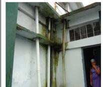
Leaking pipes and overflowing septic tank located next to kitchen area of Nongpoh DH
