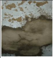
Part of ceiling has collapsed in MO's Quarter of Nonglang PHC due to seepage of water
