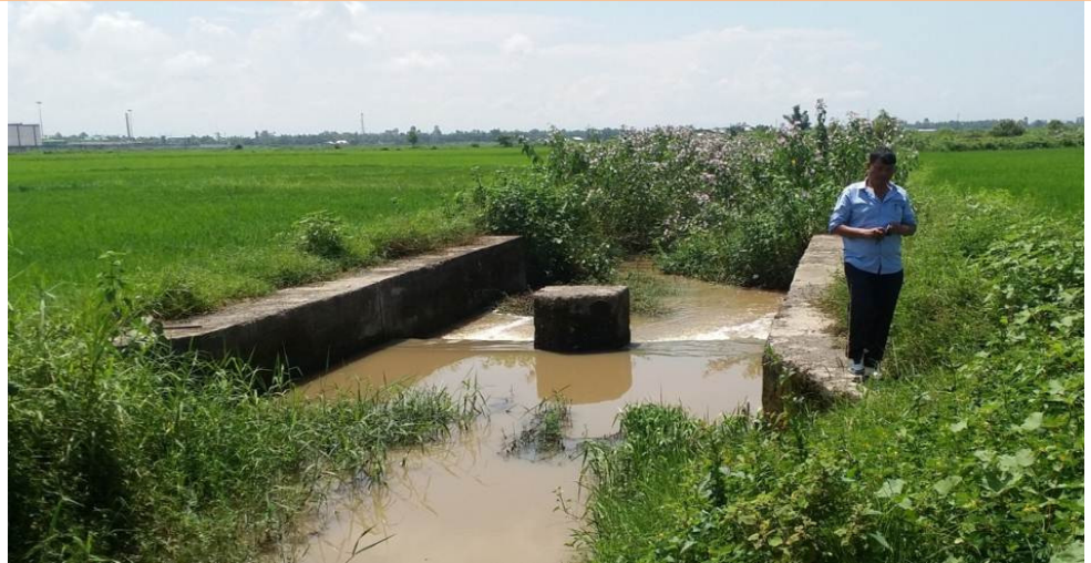
Pick-up-weir at Leima Mapa Merakhong Maril with no canal and no gate/shutter (expenditure - ₹17.44 lakh)
