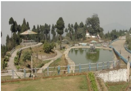
Figure 2.1: Concrete pond of Jorepokhari WLS
