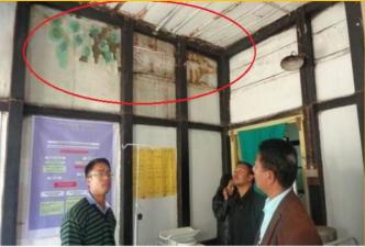
Damp labour room, PHC Tadubi functioning from the old IB constructed in 1963
