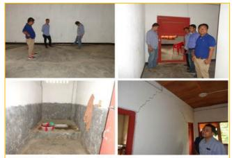
PHC T. Waichong completed in July 2012 at a cost of ₹ 59.47 lakh had developed cracks at the joining of wall and floor, crack in the ward rendering it unusable, toilet without water connection and crack on the wall
