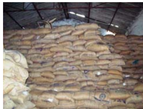
Photograph depicting inside view of Meral block godown in Garhwa district whose roof was damaged depicting plastic sheet to cover roof to protect food grains from rain water (20 August 2016)
