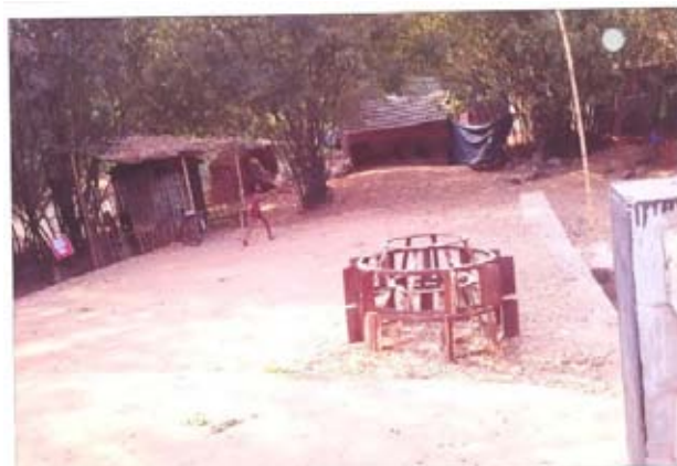
Photograph of approach road of the bridge obtained during joint physical verification
