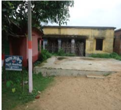
PHC & HSC, Maluti operating in one building at Shikaripara, Dumka district
