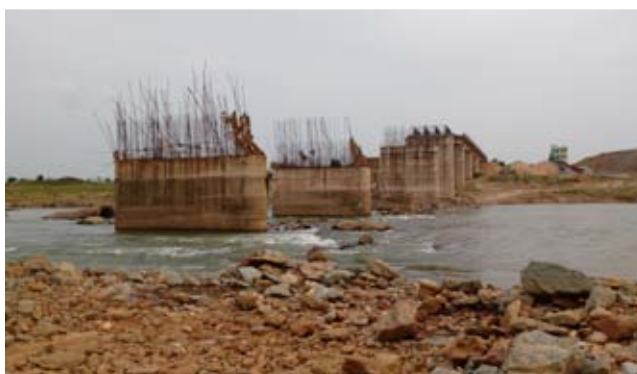
Photograph of abandoned bridge obtained during joint physical verification
