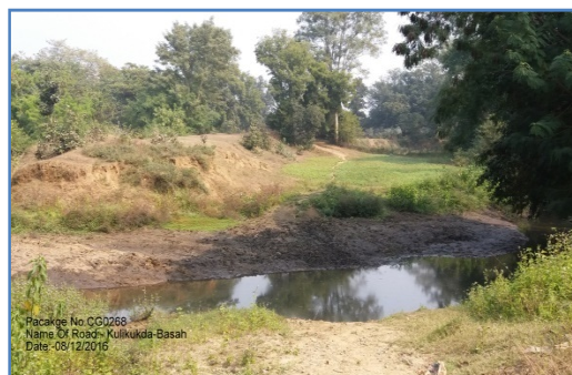
Missing link-Kulikuda to Basaha road of Bilaspur
