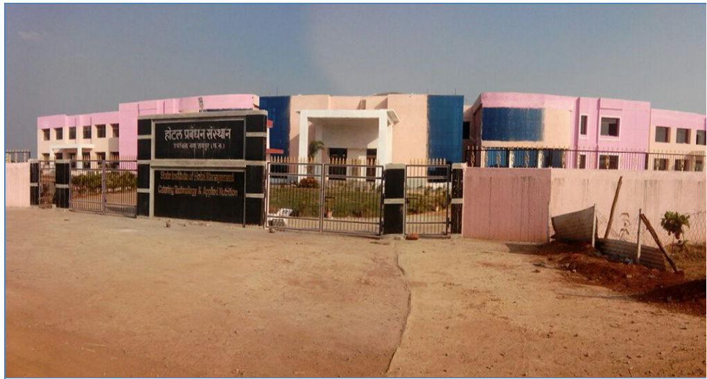
Institute of Hotel Management, Raipur not functional as on January 2017
