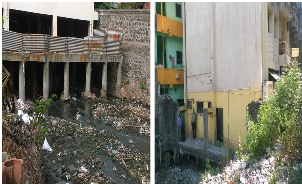
Picture 5 and 6: Unauthorised constructions
