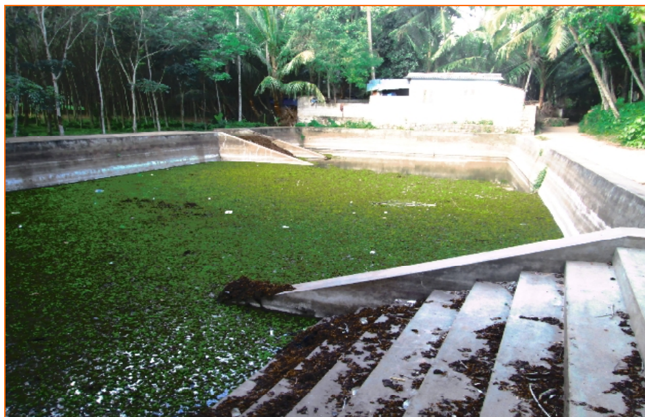
Picture 5.1: Unclean condition of Kulachavilagam Puthankulam in Ponmanai TP
