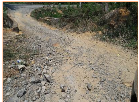
Picture 4.8: Bad condition of Kamarajar Road
