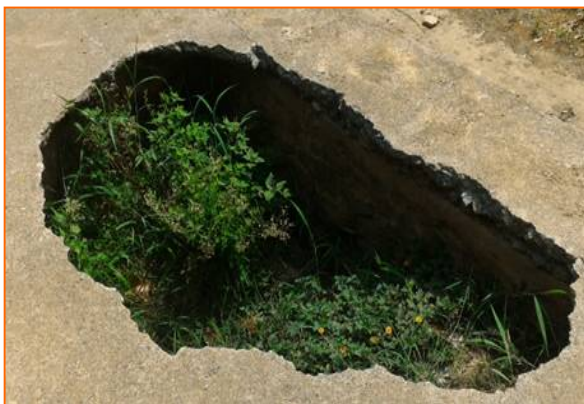
Picture 4.7: Bad condition of Pandivillai Road
