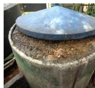
Pre-digester of 300 kg plant filled with waste in Kakkad
