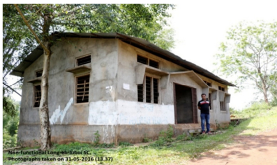
Incomplete building of Long-eh Luboi SC in Karbi Anglong (31.05.2016)
