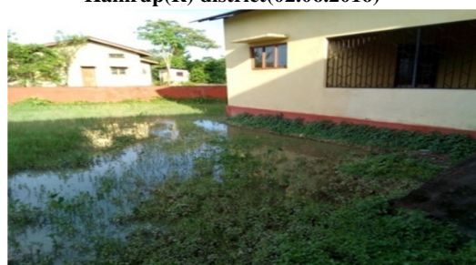
Water logging in Dakhinhengera PHC, Golaghat district (30.07.2016)
