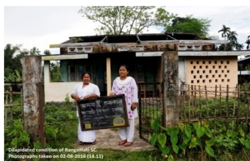
Dilapidated condition of Rangamati SC, Kamrup(R) district (02.06.2016)
