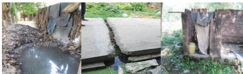
Lack of drainage system at Banbania colony
