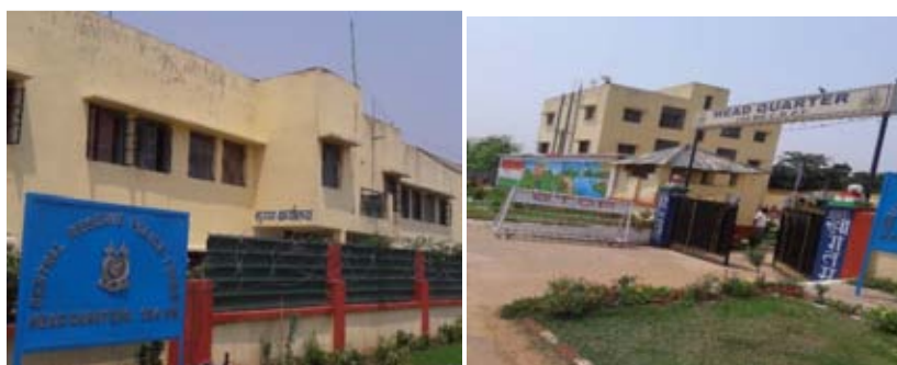
PHC, Building, Pradhankhanta (Baliapur) occupied by CRPF
