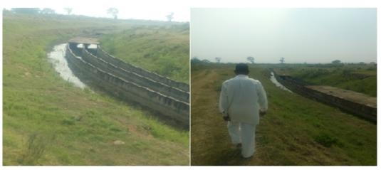
Spillage of water between Chainage 760 and Chainage 782 during Joint Physical Verification
