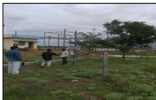
AWS (11717), Ramapur, Duvvur Mandal, Kadapa district (Andhra Pradesh) located near Chintakunta electric substation
