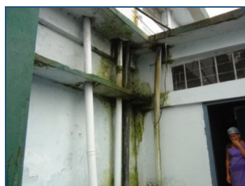
Leaking pipes and overflowing septic tank – DH, Nongpoh, Meghalaya
