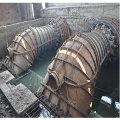
Draft tube with elbow section at Paharma SHP
