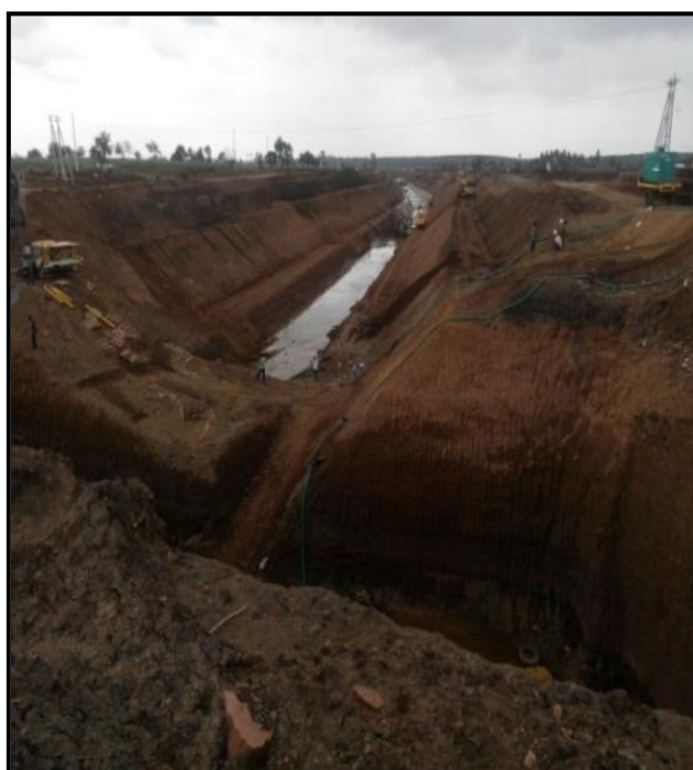
Chart No.2.1.3: Intake channel before submergence when water was at RL 507 metres (June 2016)
