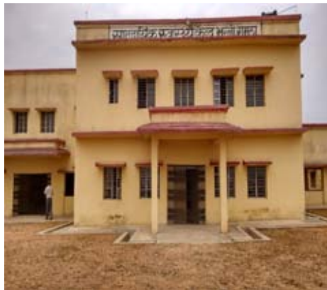
Building constructed for CHC Bharno in Gumla lying unutilised
