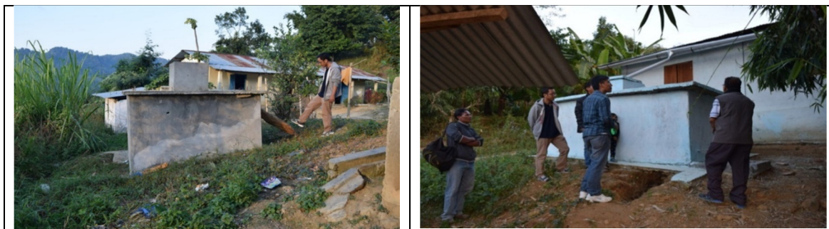
Tanks without Recharge Pits and Fencing at New Lamlo Village
