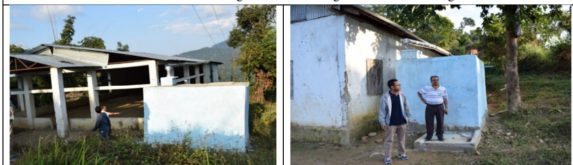
Tanks without Recharge Pits and Fencing at Notun Khheti Village
