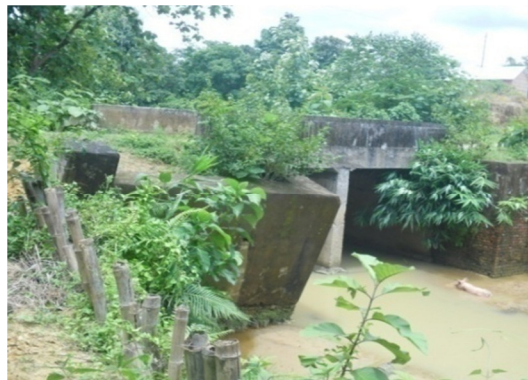
Non rectifiable damaged CD
