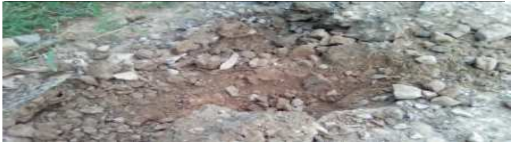
Connectivity road alongwith drains from village towards river, Nayagaon, Chandrapura (GP, Sunwas)
