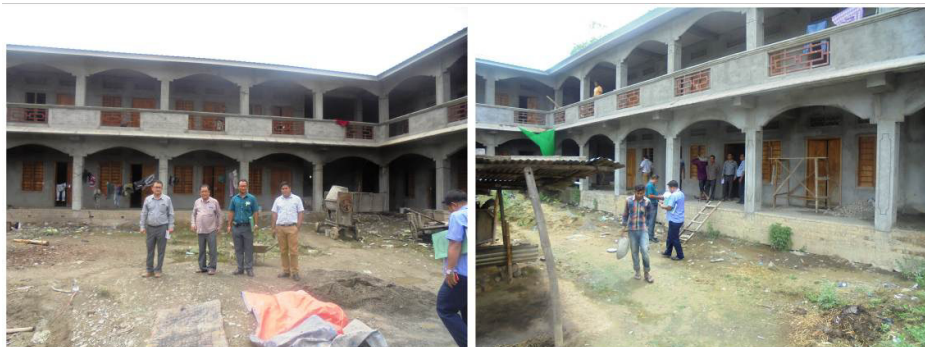
Front view of incomplete Boys hostel
