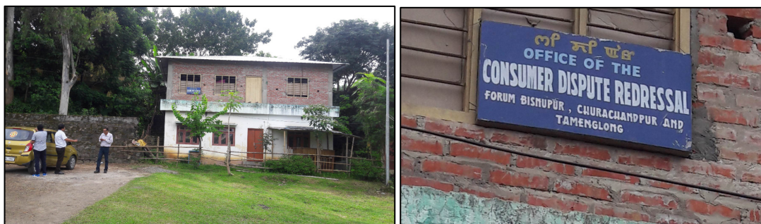
Joint Physical Verification at the stated site for Civil Defence set up in Bishnupur District. The building shown to Audit was a building of Consumer Dispute Redressal Forum, Bishnupur, Churachandpur and Tamenglong districts
