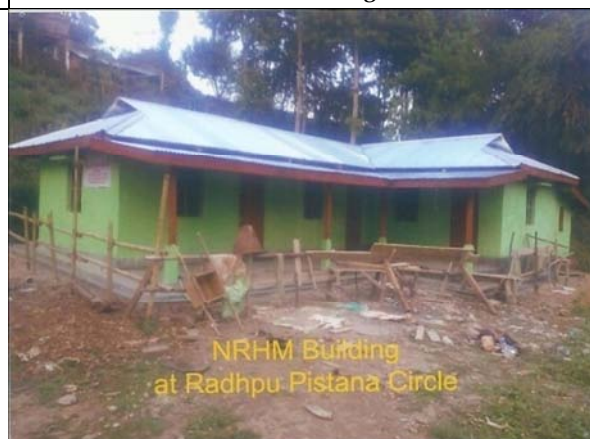
Unoccupied Sub Centre building at Radhpu, Lower Subansiri
