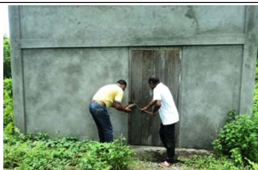
Non-functional plant was installed in this shed at General Hospital, Tezu.
