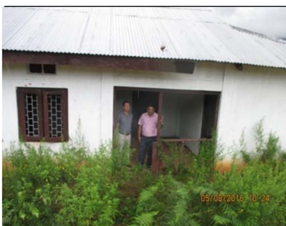
Unoccupied Sub Centre building at Khodaso, East Kameng
