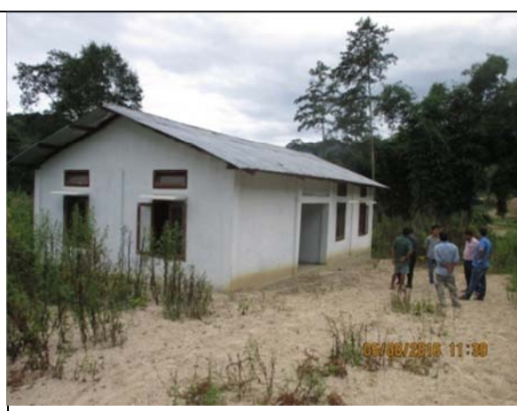
Unoccupied Sub Centre building at Alangtopte, East Kameng
