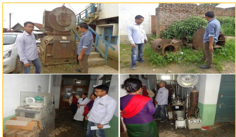
Uninstalled and parts of Incinerator, unused Baby incubator and Autoclave and Suction Machines at District Hospital, Ukhrul
