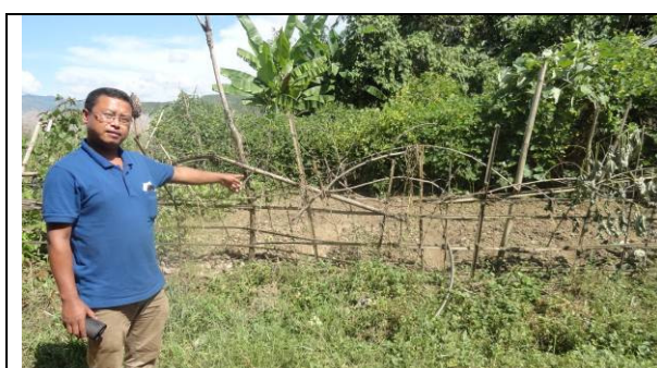
Site for Building of Island AWC, Machi Project in Chandel district which was listed as constructed in Phase-II.
