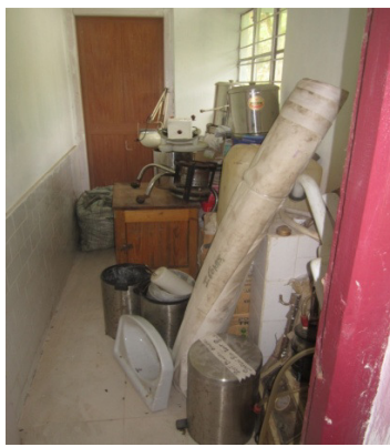
Toilet outside female ward in Riango CHC used for storage
