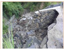
Pucca Dam across Vaipal stream - damaged left side wall and downstream cut-off wall
