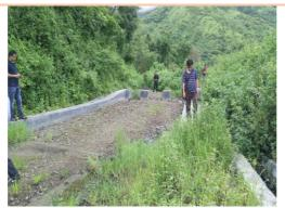
Pucca Dam at Chihjang - Fully silted upstream and downstream. Water not available at the source
