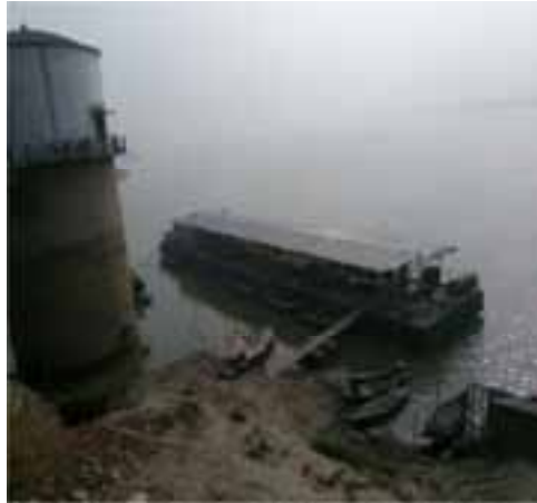
Floating jetty of Munger PWSS
