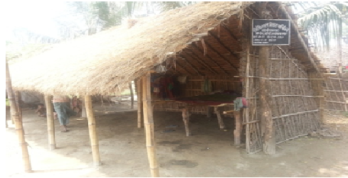
AWC running in temporary shed without toilet, kitchen, water facility (Koylasthan, Mahishi Saharsa).
