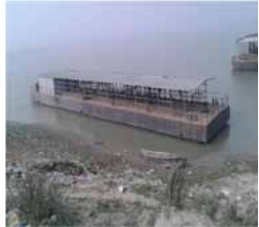
Floating jetty of Jamalpur PWSS
