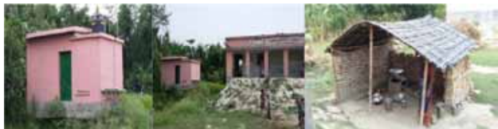
Kitchen constructed without any road connectivity at Primary School Ramnagar Math, Khanpur, Samastipur and therefore MDM was being prepared under thatched roof.
