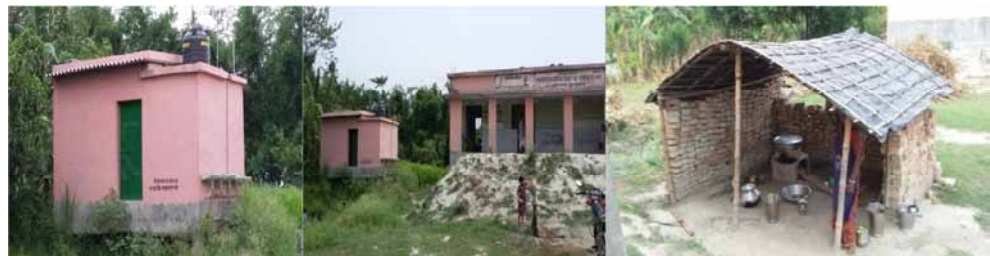
Kitchen constructed without any road connectivity at Primary School Ramnagar Math, Khanpur, Samastipur and therefore MDM was being prepared under thatched roof.
