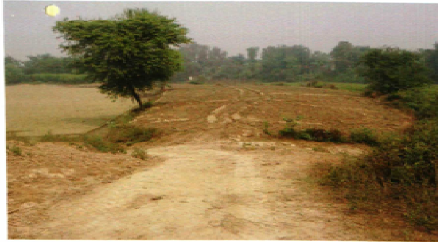
Unconstructed portion of KTP at 29.20 KM
