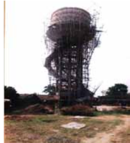
Under construction elevated service reservoir of multi-village PWSS of Sultanganj and Nathnagar block of Bhagalpur district
