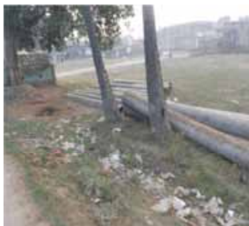
Pipes related to Maner block of Patna district laying scattered in the field
