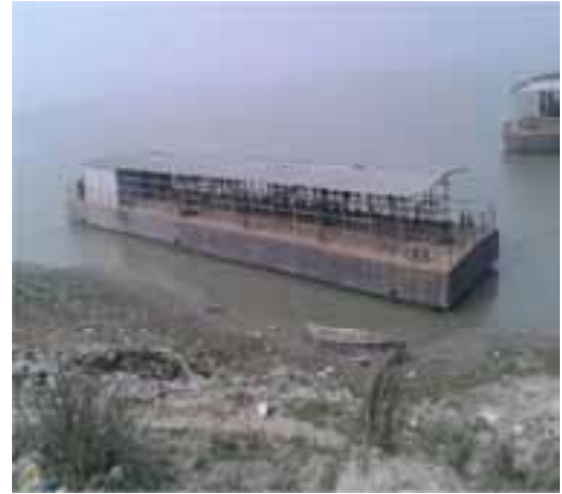
Floating jetty of Jamalpur PWSS
