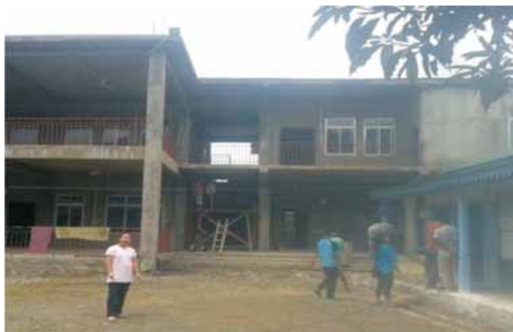
SDH Khawzawl under construction
