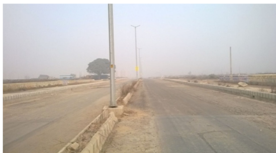
Rohini Zone: Construction of Main carriageway
