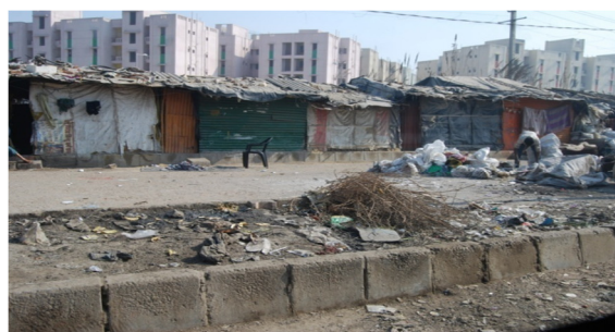
North Zone: Construction of Peripheral S.W. Drain & culverts in Sector G-7 & G-8
