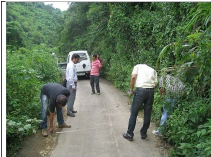
Imphal East: Construction of Road from Luwangsangbam Jn. To Kameng (MN0420) Deficiency in carriageway width i.e. 2.7 m from ch. 3.20 km to 4.70 km
