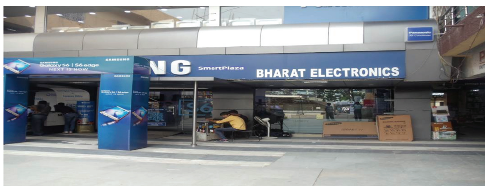
Encroachment of common space at BirsaVihar Market complex, Ranchi
