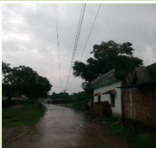
Non-construction of side drain in Baidynathpur to Bahadurpur in Deoghar district, Jharkhand
