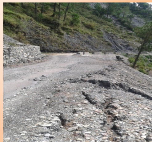
Unpaved and without revetment of Rumehar-Lam road in Kangra district, Himachal Pradesh
