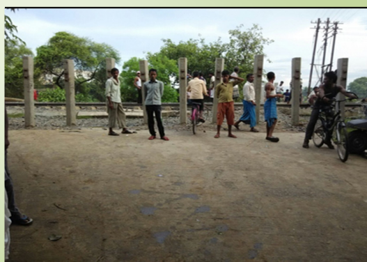
Connectivity was not provided to habitation because road was blocked by cement concrete pillars on both sides of railway track (in package no - BR-06R-148, Bhagalpur district, Bihar)
