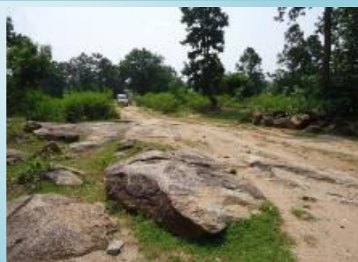
Hard rock and forest land lying in path of the road 'L059-REO main road Kutmakachhar to Murambatoli via Jhimari 'in Simdega district, Jharkhand
