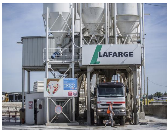
Lafarge Cement Factory
