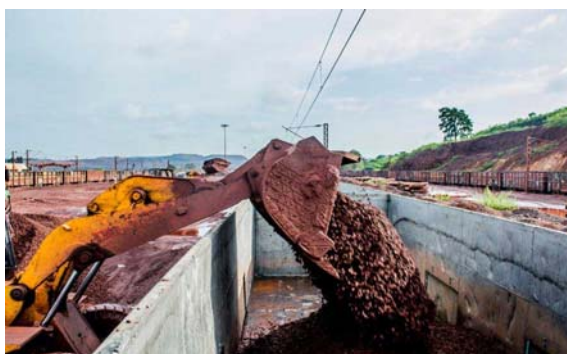
Land encroached by Railway
