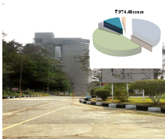
Jojobera Cement Plant, Jamshedpur
