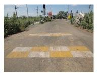
provided on all LCs over the total width of the road with proper road warning signs. Till such time these are replaced with rumble strips of proper design by the Road authorities, as a temporary safety measure, Railways were to provide speed breakers.
