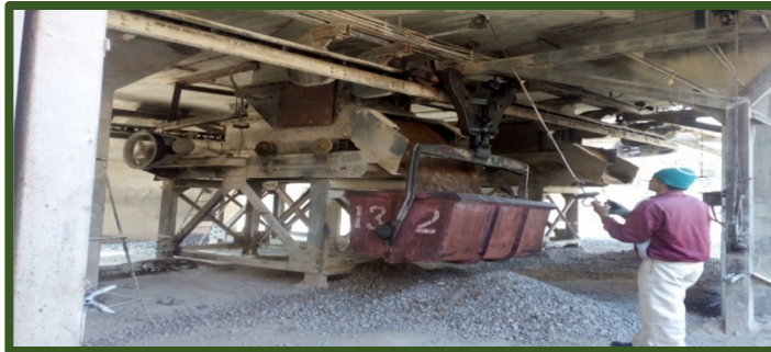
Workers working without personal protection equipments in Manal Lime Stone Mining Project, Himachal Pradesh
