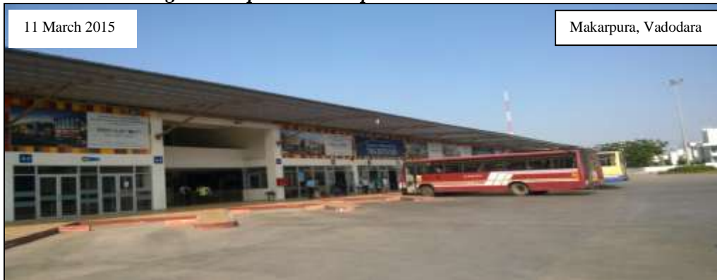
Picture 4.5 Showing the completed Makarpura Bus Station at Vadodara
