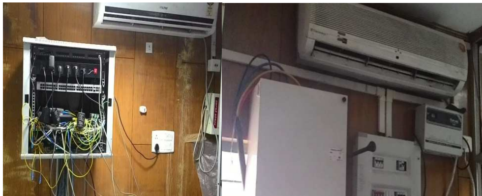
Central Data Centre (Kar Bhavan, Dispur) (4 June 2015)
