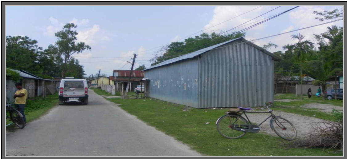
Construction of classroom of Kalgachia Girls ME School with roofing sheets instead of brick wall as per sanctioned Plan and Estimate in Jania LAC under MLAADS 2012-13 (28 April 2015)
