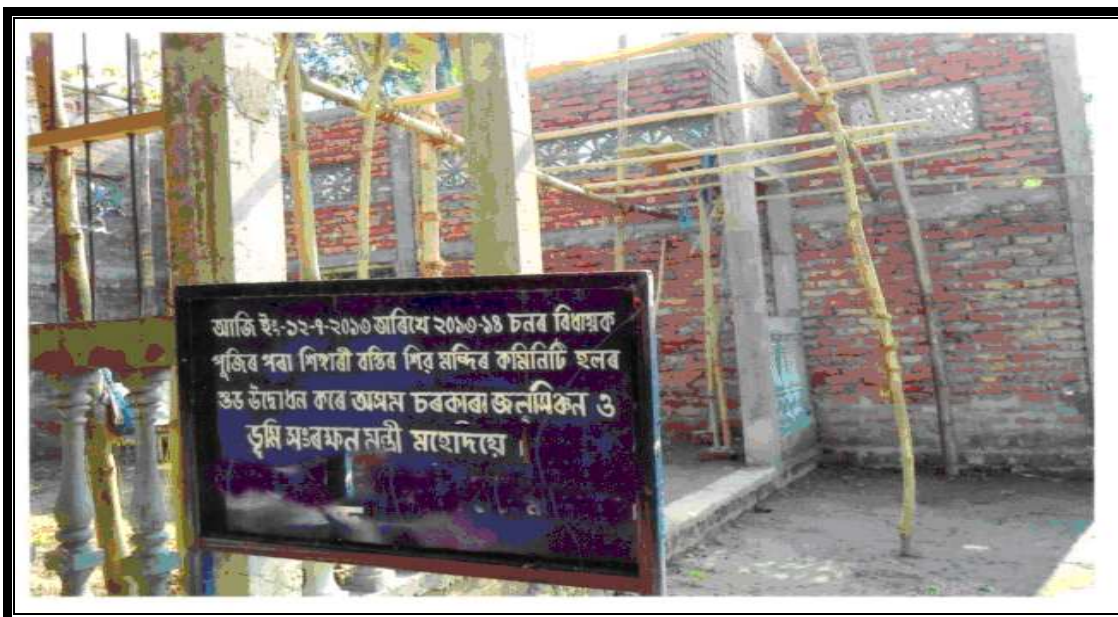
Incomplete community hall building inaugurated by the MLA of Hojai LAC of Nagaon district (08 May 2015)
