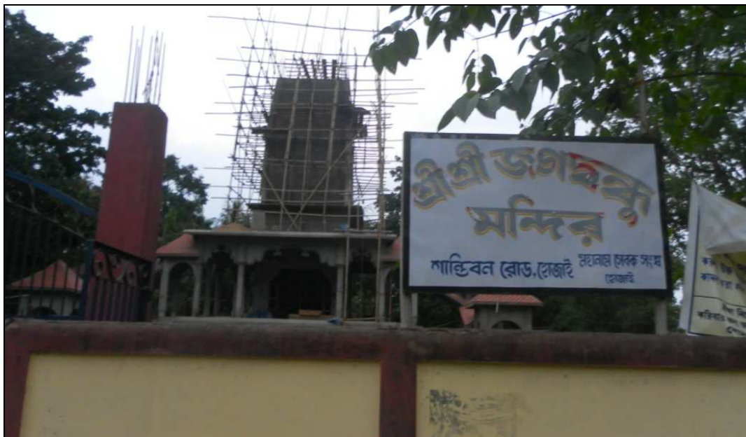
Construction of Jagat Bandhu Mandir at Hojai Town, Ward No .8 under MLAADS 2013-14 (21 May 2015)
