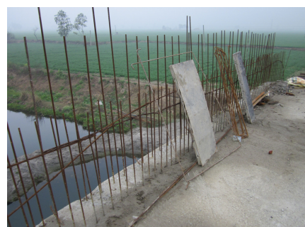
Incomplete bridge (on 14-01-2016)
